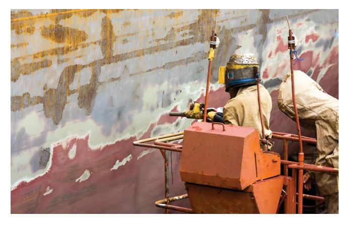
The ABS Hull Inspection and Maintenance Program (HIMP) was designed to help shipowners and operators effectively inspect and maintain the hull structures on their vessels. HIMP inspections help shipowners systematically identify, record, examine, and grade hull structure conditions, including defects.
