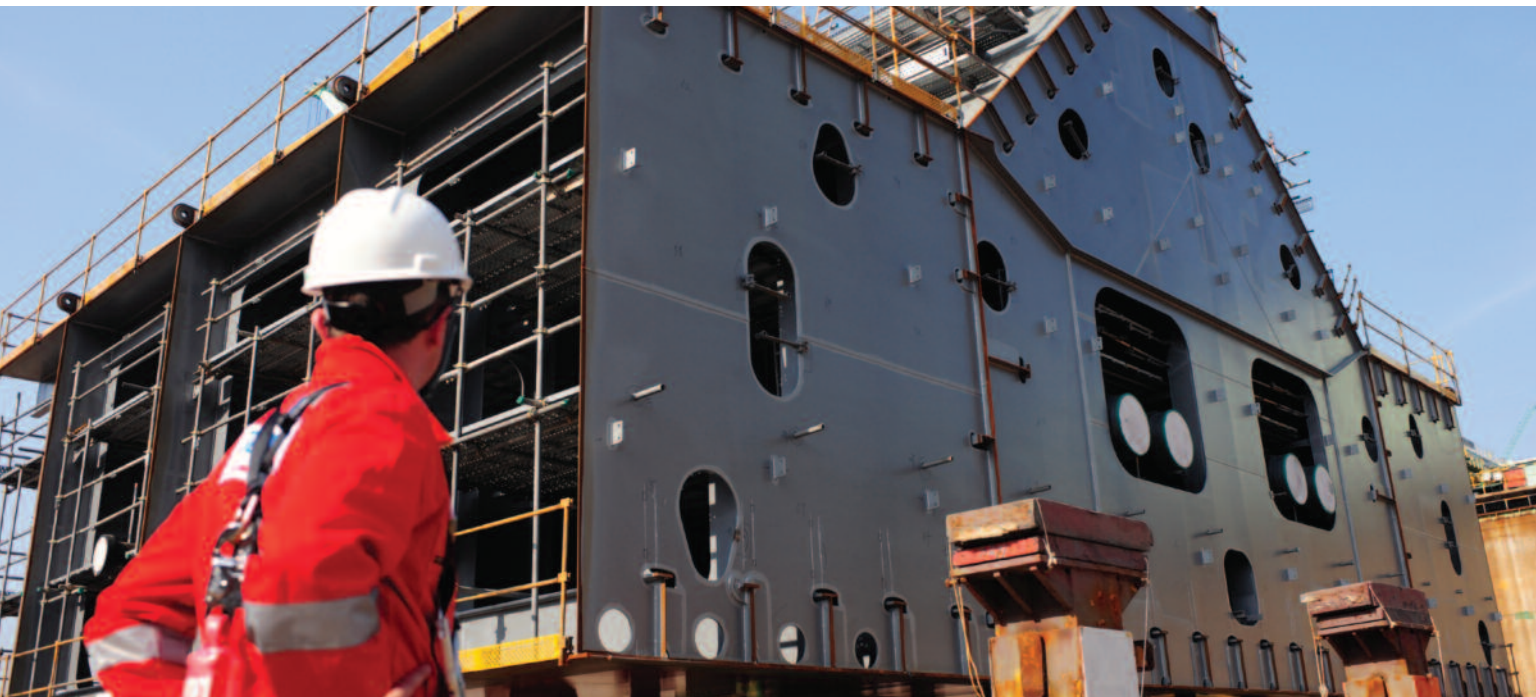
The LNG and natural gas liquids will be stored in tanks in the hull. (Image courtesy of Shell)
