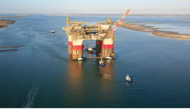
The deck box hull will support the topsides production facility configured into modules fabricated and lifted independently. The topsides modules will house production, compression and power generation equipment, with provisions for future production, water injection and additional power systems.
