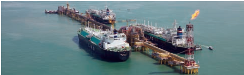
ABS has classed Petronas' Melaka Terminal, which employs an older MISC LNGC as a storage unit connected to a regasification unit on the jetty.
