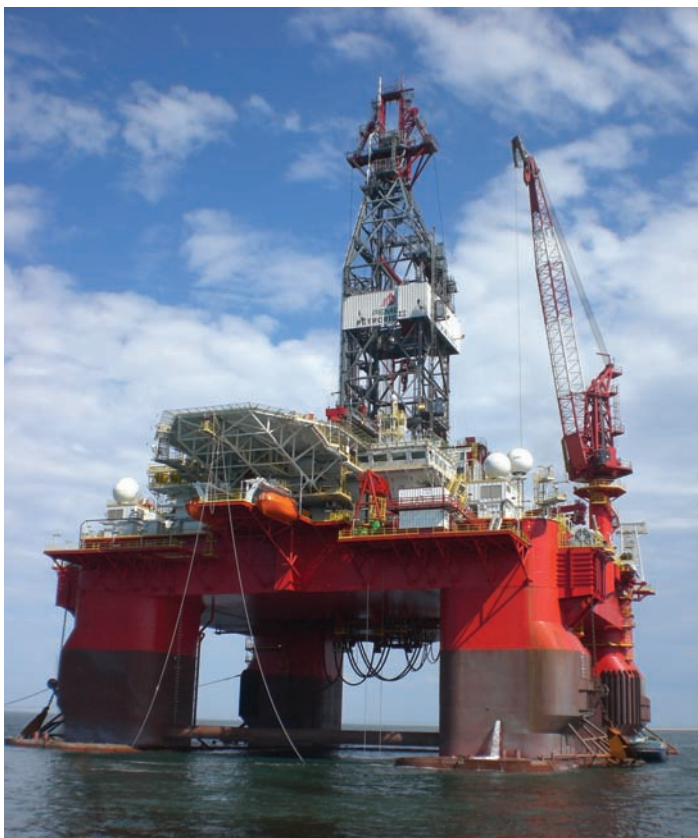
Classed by ABS, PEMEX's Centenario GR is a sixth-generation DP semisubmersible capable of drilling in 3,000 m (10,000 ft) water depth. (Photo courtesy Grupo R)
