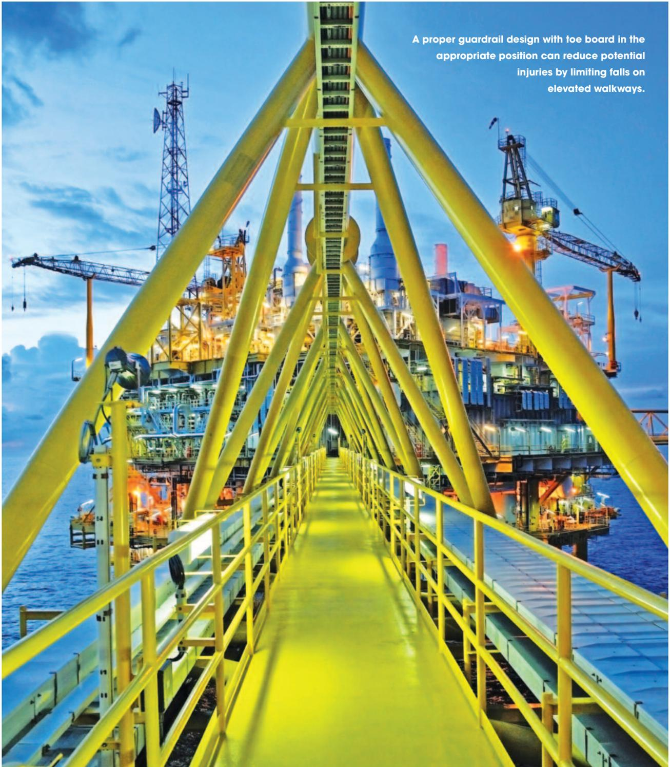
A proper guardrail design with toe board in the appropriate position can reduce potential injuries by limiting falls on elevated walkways.
