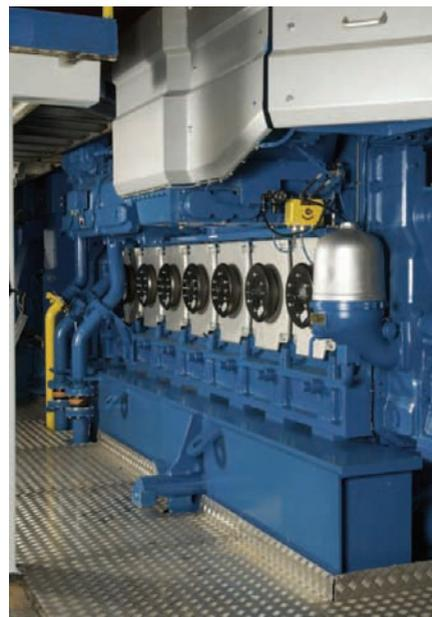
The Wärtsilä 6L34DF dual-fuel technology provides 100% redundant backup should a switch from one fuel to another occur without any interruption in power generation. (Photo courtesy Wärtsilä)
