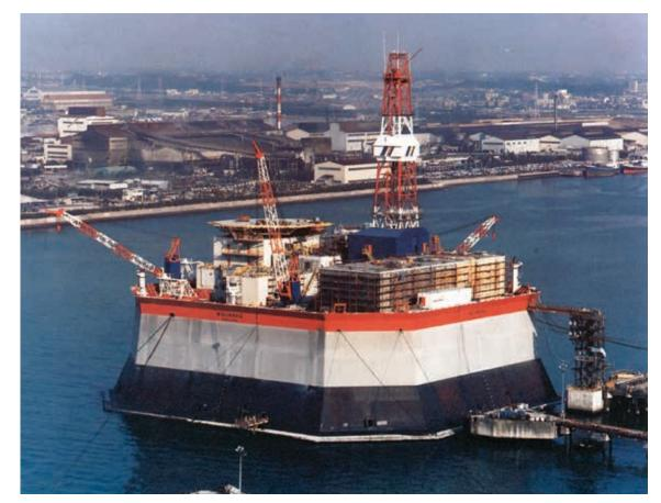
The steel-encased Arctic drilling rig MOLIQPAK, built to ABS class in 1984 for exploration in the Beaufort Sea, was refitted under ABS class for service in Russia's Sakhalin I Field in 1999.
