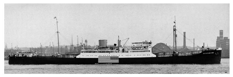
The twin-screw, diesel powered CITY OF NEW YORK was a passenger liner built in 1930 by Sun Shipbuilding & Dry Dock Company for American South African Lines.
