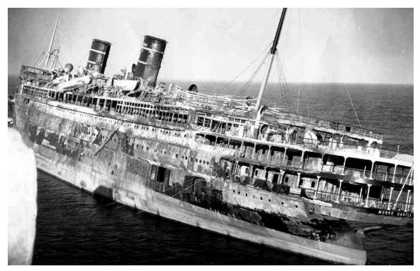
On 8 September 1934, the SS MORRO CASTLE caught fire and burned, killing a total of 137 passengers and crew members. The devastating fire was a catalyst for improved shipboard fire safety. Today's requirements for using fire retardant materials, automatic fire doors, ship-wide fire alarms and increased attention to fire drills and procedures resulted directly from the disaster.
