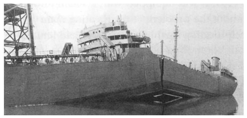
The SS SCHENECTADY was a T2 tanker constructed by the Kaiser Shipbuilding Company in Portland, Oregon. The keel was laid on 1 July 1942, the completed hull launched on 24 October, and the vessel was completed on 31 December. However, on 16 January 1943, shortly after returning from sea trials, the hull cracked almost in half, just aft of the superstructure. ABS had a lead role in the investigation to determine the cause of the fracture and to develop a solution.
