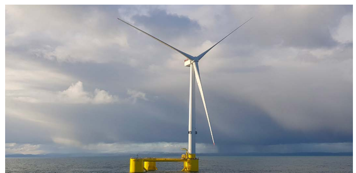
Kincardine: ABS-classed and the world's largest floating offshore wind farm when installed.
