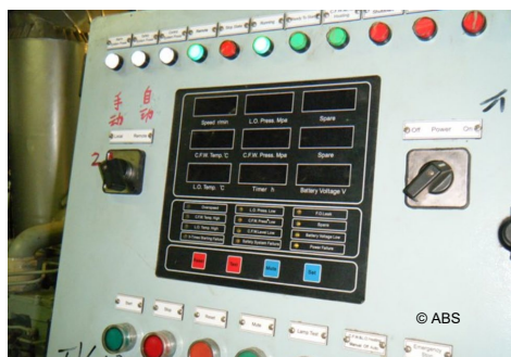
Emergency generator control display not working due to faulty PLC card
