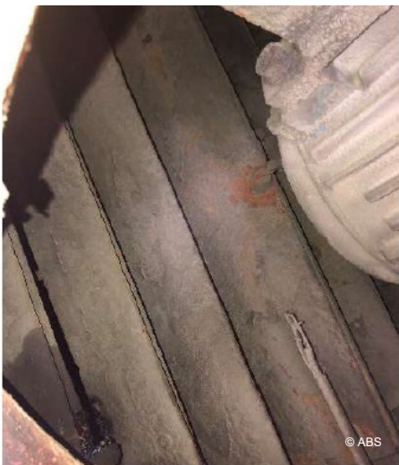
Fire damper not fully closing – before
