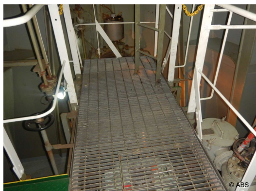
Steel gratings in way of propeller shaft in the engine room were properly secured
