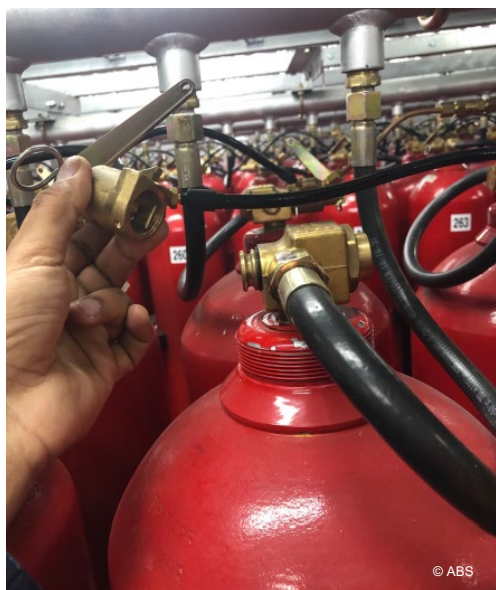
CO 2 bottle heads found disconnected
