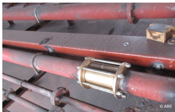
Leaking fire line expansion bellows replaced
