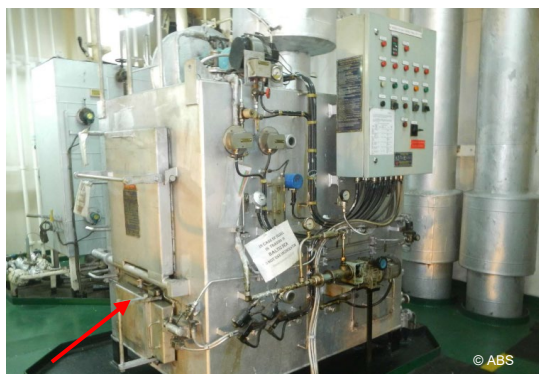
Packing for the incinerator door renewed
