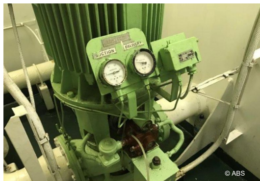
Emergency fire pump running after repair
