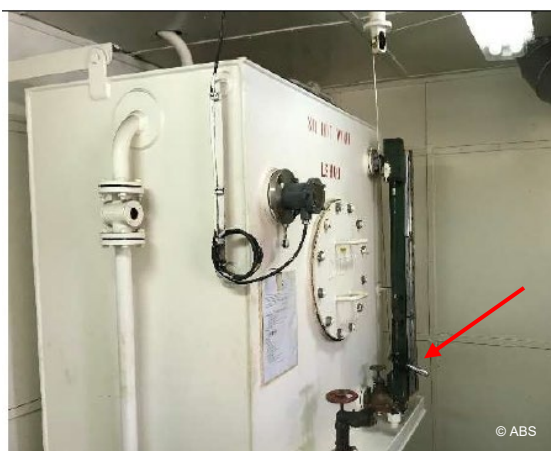
Emergency generator quick closing fuel valve found inoperative
