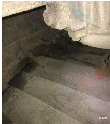
Fire damper fully closing – after
