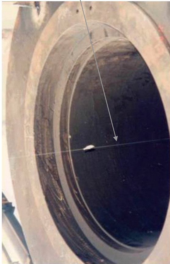
FIGURE 2 Piano Wire Application
