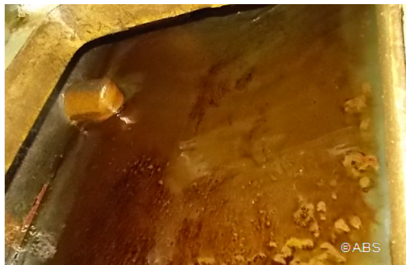
Sign of oil sheen in auxiliary engine fresh water expansion tank
