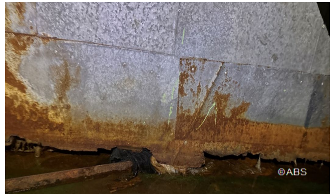
Air conditioning and heating system enclosure wasted
