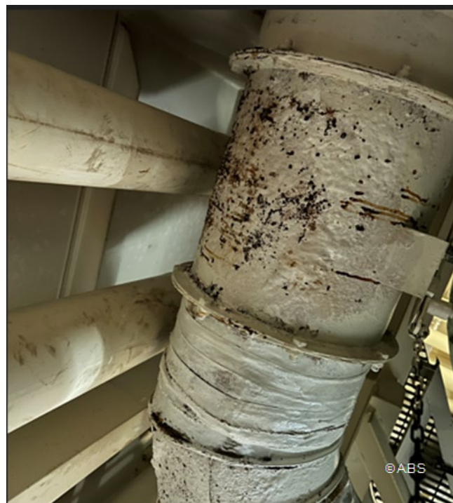
VENTILATION DUCT IN ER HOLED AND COVERED WITH TAPE
