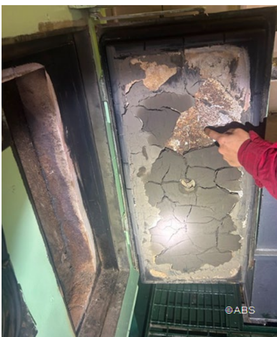
INCINERATOR DOOR REFRACTORY MATERIAL DISINTEGRATED DUE TO AGE AND HEAT
