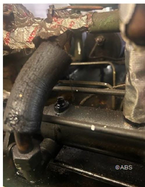
INCINERATOR FUEL OIL PIPE WITH MISSING INSULATION AND LEAKING FUEL PUMP
