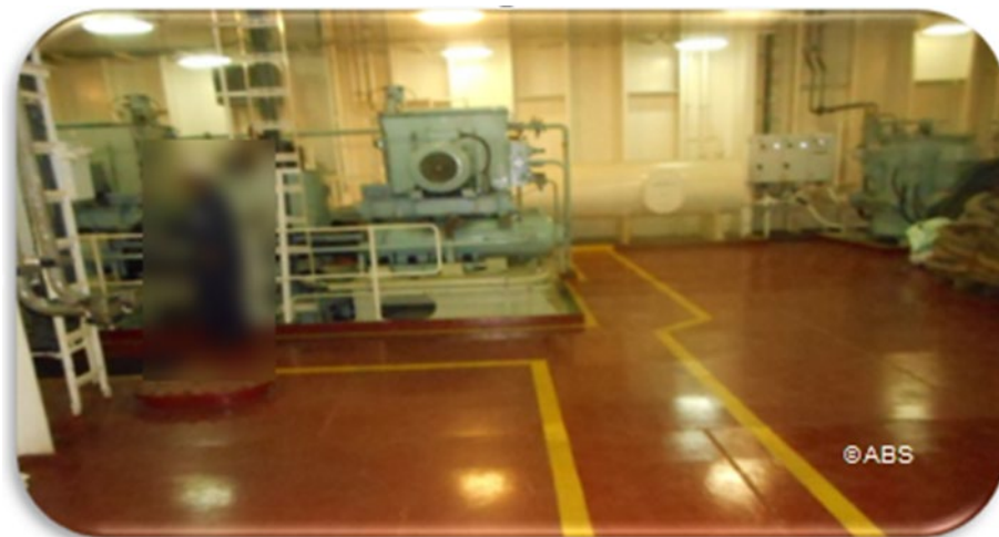
STEERING GEAR ROOM WITH MISSING HANDRAILS, GRATINGS OR OTHER NON-SLIP SURFACE TREATMENT AS REQUIRED BY SOLAS REGULATION II-1/29.13 AND CLASS RULES MVR 4-3-4/1.7
