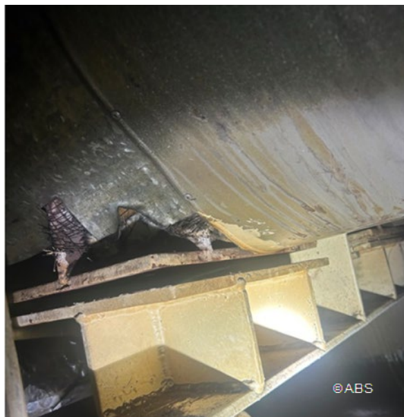
EXHAUST GAS PIPE NOT SUPPORTED BY ITS FOUNDATION
