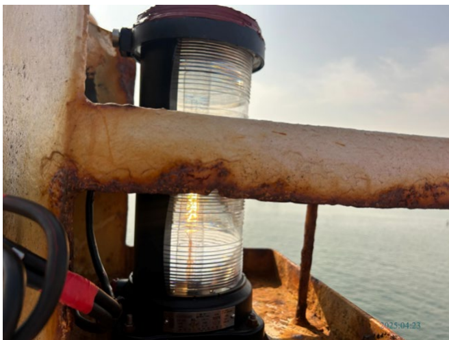
The horizontal light arc of mast light on top of the forecastle not complying with requirements of COLREG.
