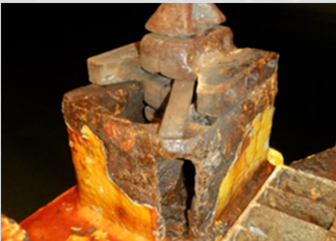
Twist lock foundation at container housing cracked
