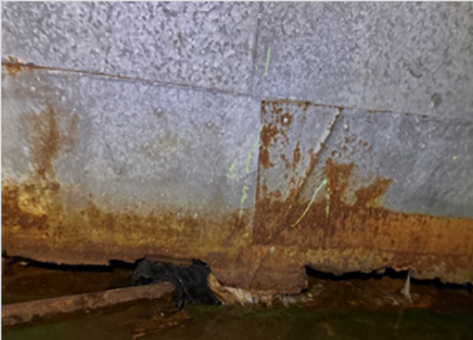
Air conditioning and heating system enclosure wasted
