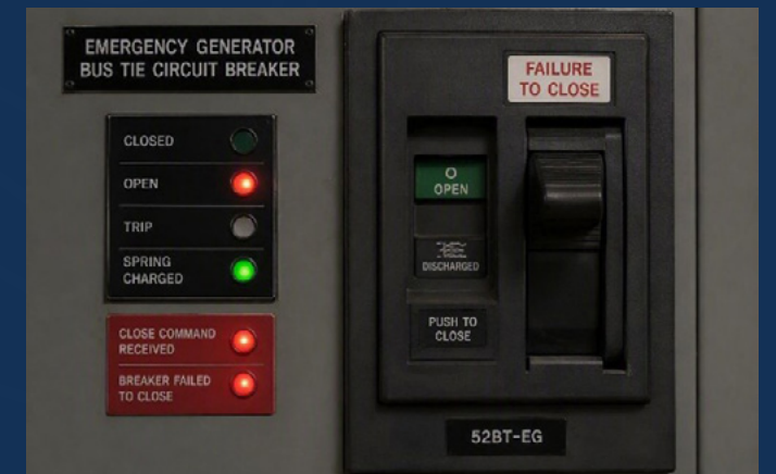
Figure 3: Emergency generator is unable to connect to the emergency switchboard at the time of the operational test.
