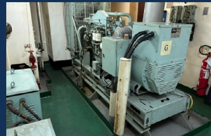
Figure 3: Emergency generator is unable to connect to the emergency switchboard at the time of the operational test.
