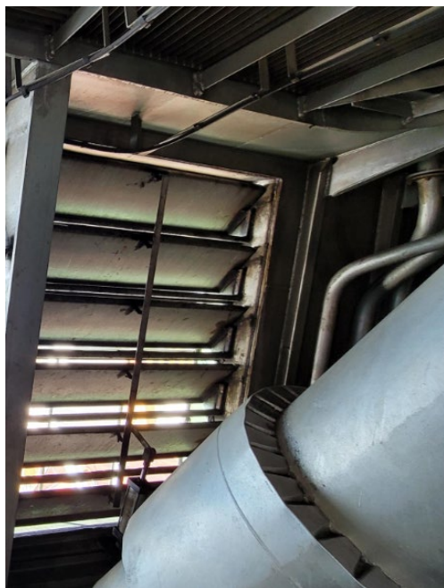
Fire damper not fully closing – before
