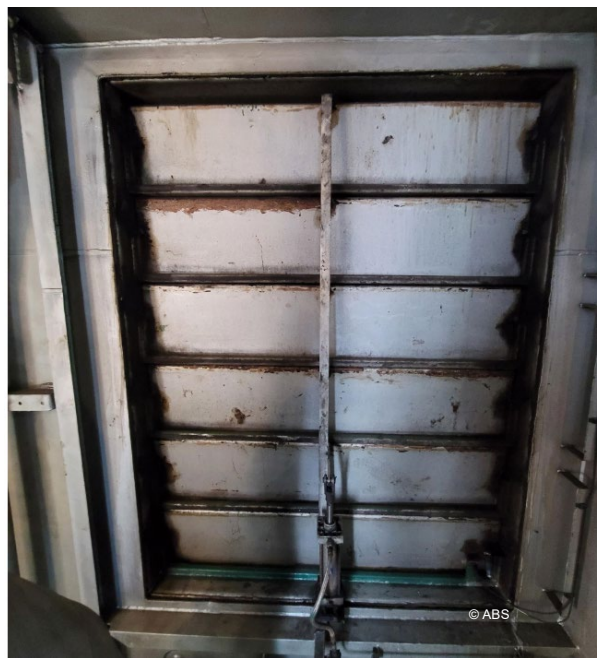
Fire damper not fully closing - after
