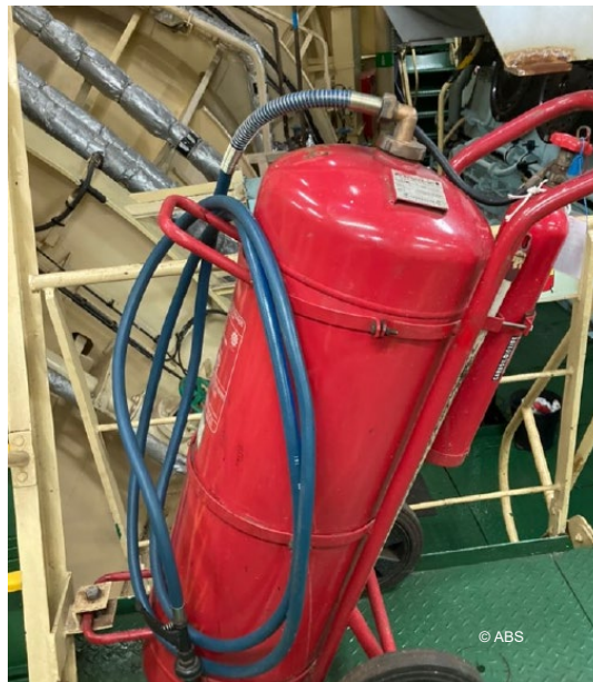
Portable extinguisher flexible hose cracked - after
