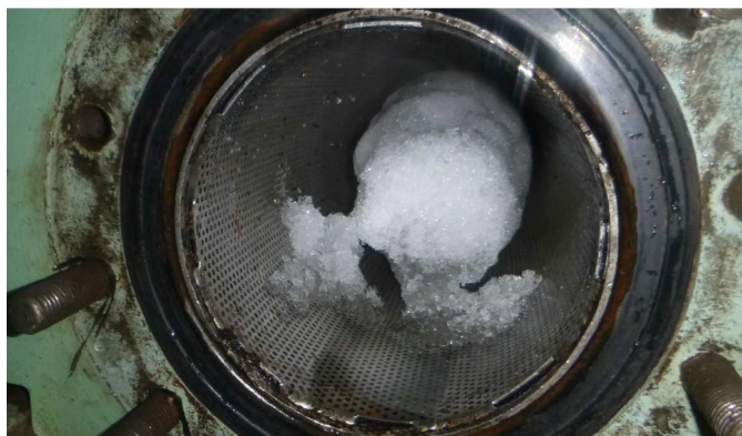
Overheating due to high temperature of main lubrication oil caused by strainers/filters in sea water cooling line blocked with ice - before
