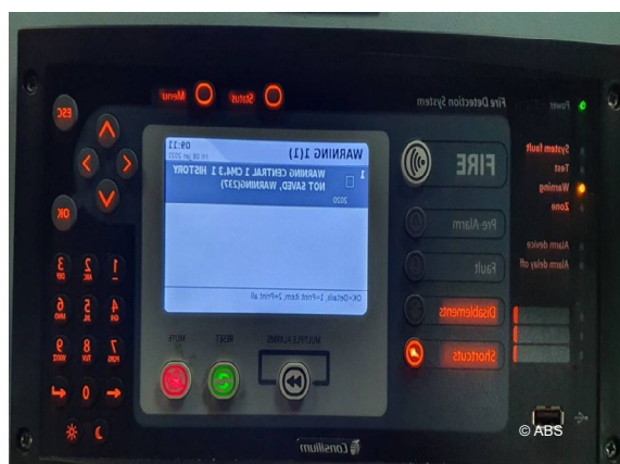
Fire alarm fault
