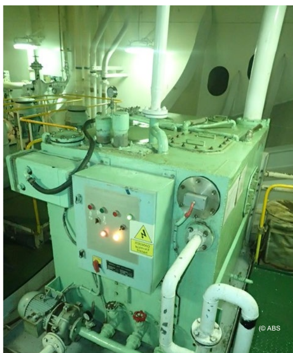
Sewage treatment plant not operational
